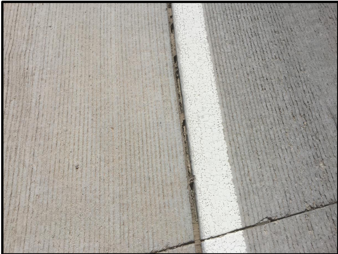
Figure 8 – Joint sealing and gapping
