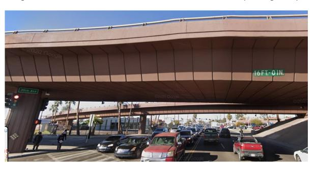
Figure 8 – Posted Minimum Vertical Clearance Indian School/US 60 Ramp Connections (Looking North)
