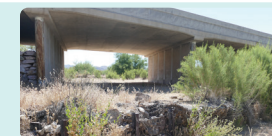
Removing the failing existing rail bank cut-off wall will result in long-term scour to reach equilibrium slope.
