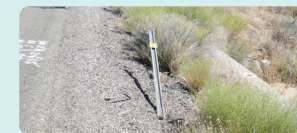
Existing culvert headwall with a damaged hazard marker within the clear zone.
