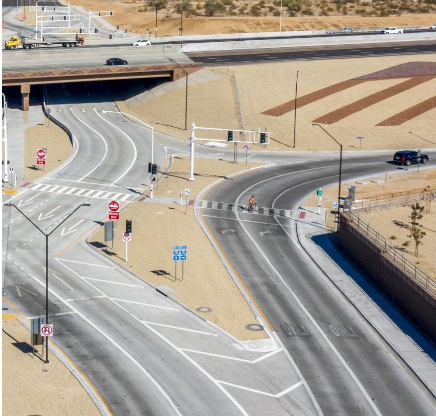
Figure 19. Signalized Channelized Right-Turn Lane at I-10 and Watson Road
