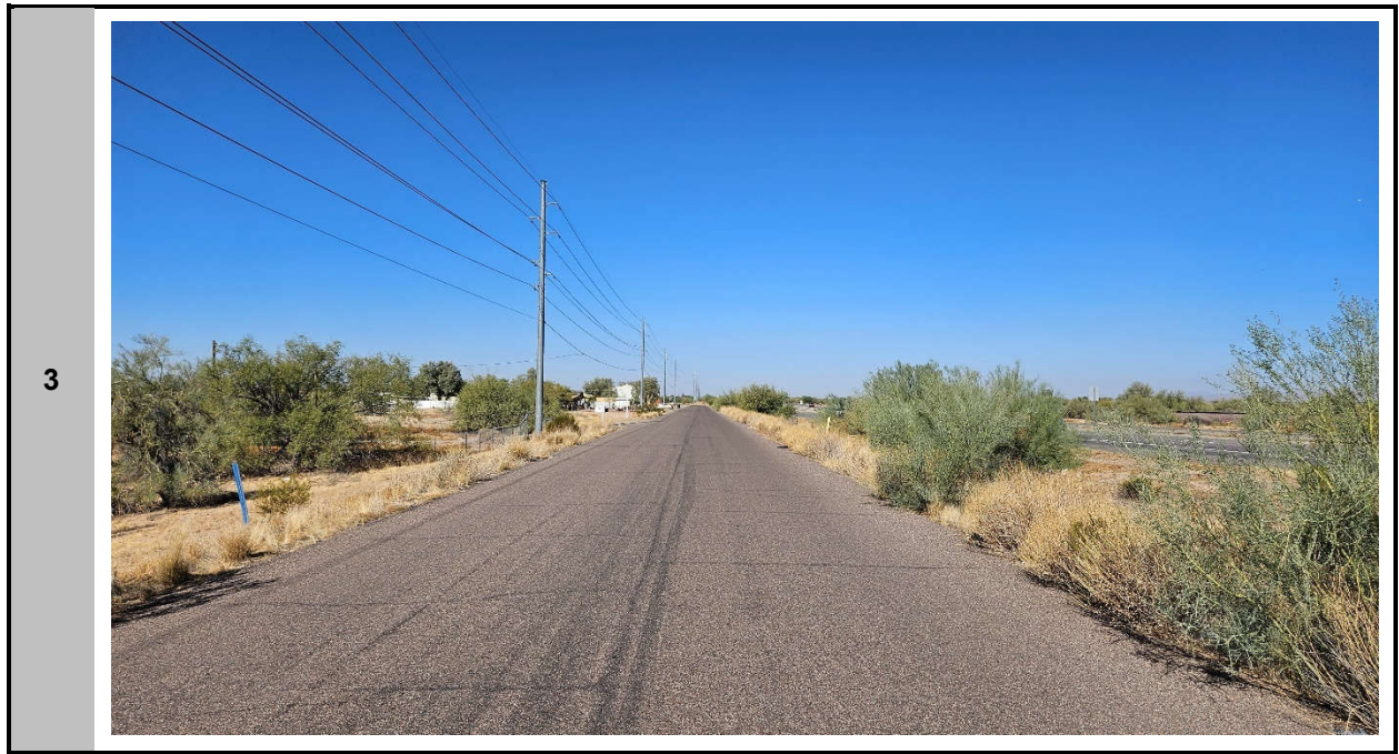
View northwest along the Grand Avenue frontage road
