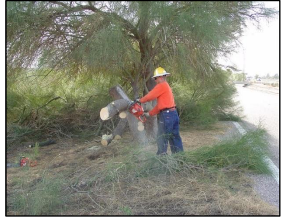
ADOT employee with proper PPE using chainsaw to remove large limb
