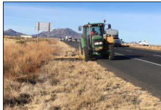
Mowing the roadway edge can reduce fire fuels and wildlife grazing.
