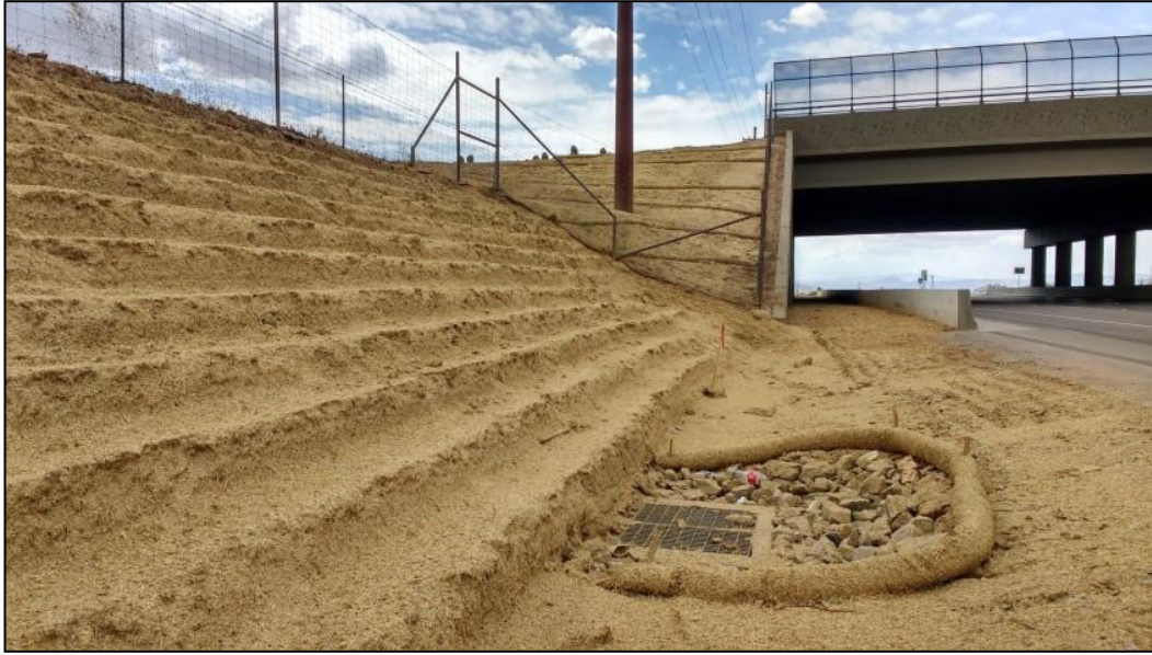
Hydrostraw mulch and tackifier applied to slope
