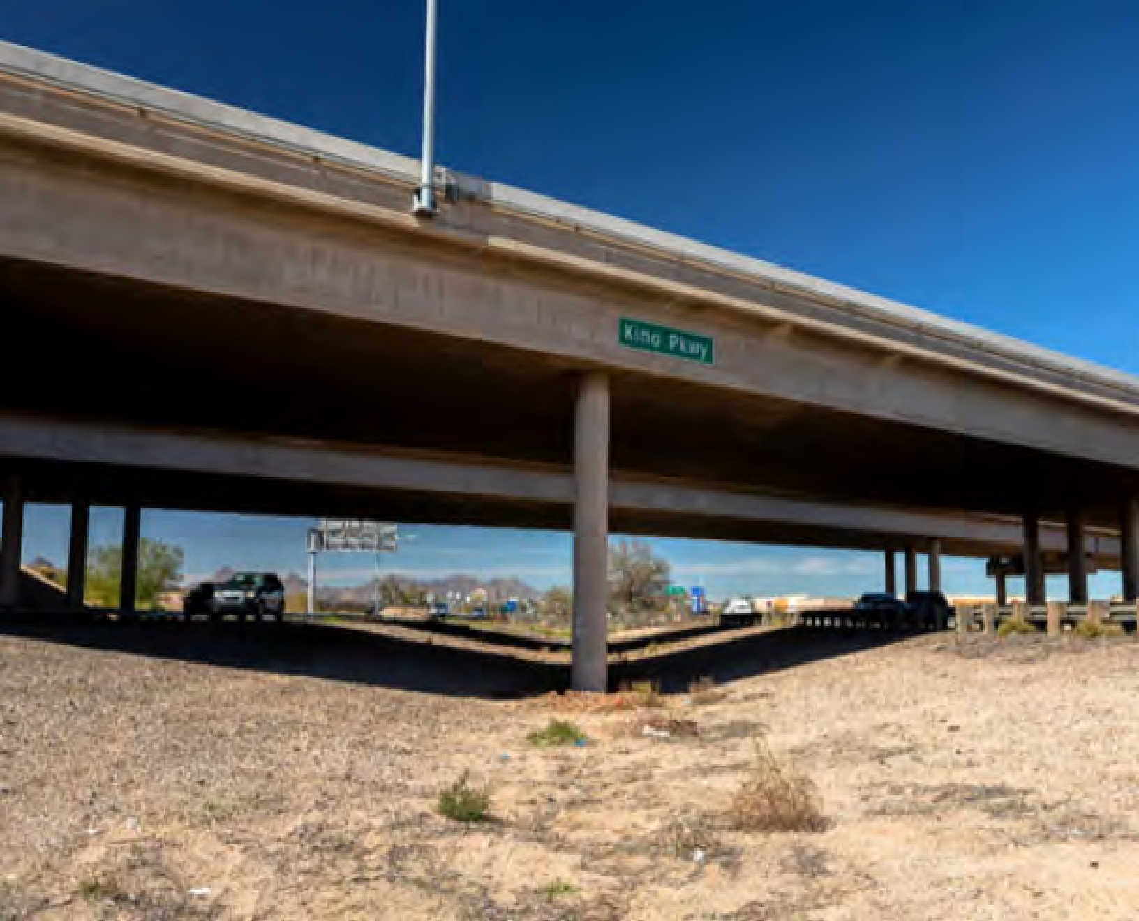
Kino Parkway overpass on I-10 in Tucson
