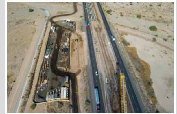
I-10: Gila River Bridge
