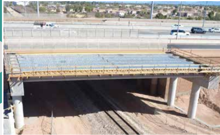
Loop 202 (Santan Freeway): Loop 101 to Val Vista Drive
