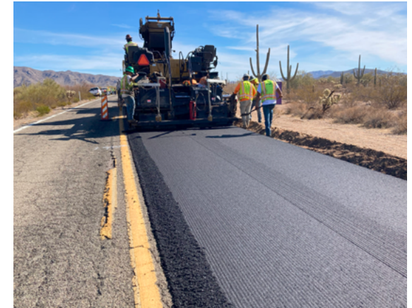
Unit 4592 Paving SR 86 MP 80 to 90
