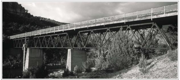
Figure 11. Black River Bridge (03128), 2002. (Trusses shown are replacement spans, erected in 1929 over original concrete piers).
