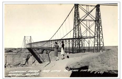
The canyon at this location was both wide and deep with steep-sided walls, requiring a single-span structure that could be erected without falsework. To solve the problem, Midland Chief Engineer W.H. Code designed this 660-foot-long steel suspension structure [Figure 43].
