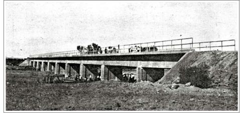
This star-crossed structure began to fail almost immediately, revealing a dangerous and expensive weakness of the state's large concrete spans. These structures were demonstrably stronger and more stable under load than their steel truss Their counterparts. poured-in-place superstructures could carry traffic well enough, but
