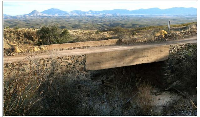
Figure 36. Black Gap Bridge (08534), a rail top concrete slab built in 1920-1921 by convict laborers. 2018.
