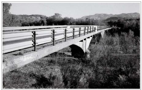
Figure 41. Kelvin Bridge (08441), 2002. (Original concrete balustrades have been replaced with Thrie beams.)
