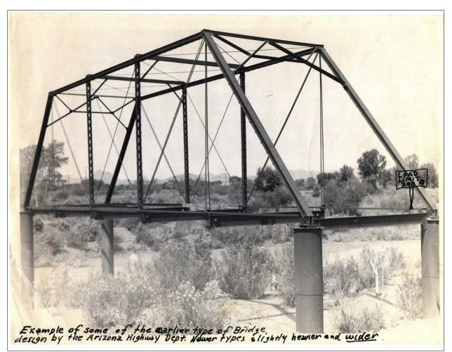
Figure 5. Unidentified pin-connected Pratt through truss, n.d. ADOT. (Bridge has been demolished.)
