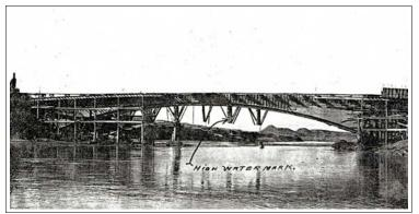
Figure 38. Holbrook Bridge under construction, showing flood damage, 1916
