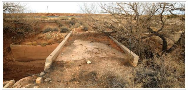
Figure 18. Jacks Canyon Bridge, 2018. (Bridge has been closed to traffic, and the steel pipe guardrails have been removed.)
