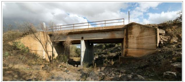
Figure 54. Cordes Bridge (08249), 2018. (The center-span pier has recently been added.)
