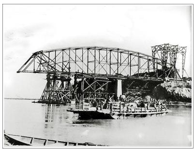
Figure 44. Ocean-to-Ocean Bridge under construction, March 1915. Arizona State Archives.
