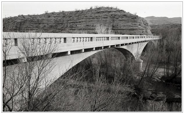
Figure 40. Gila River Bridge (08152), 2003. (The bridge has been rehabilitated, with many of the cast concrete balusters replaced.
