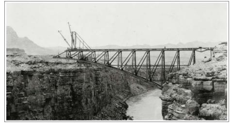
Figure 77. Navajo Bridge, last panel of south arm under construction, 1928. Library of Congress.
