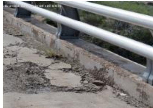
Figure 3-7 | Scaling on a Bridge Deck
