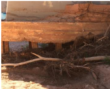
Figure 3-6 | Scour at a Bridge Pier
