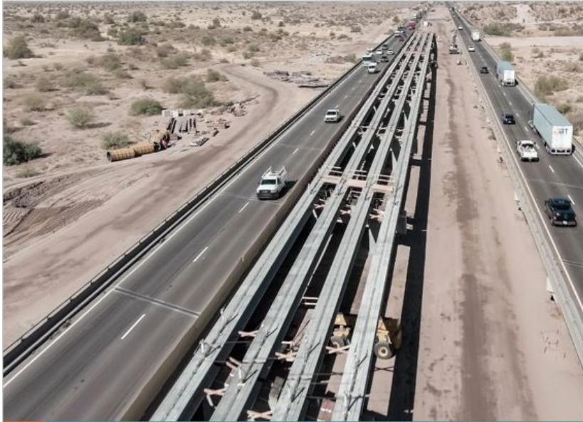
Construction of bridge girders for the Gila River on I-10 in Pinal County
