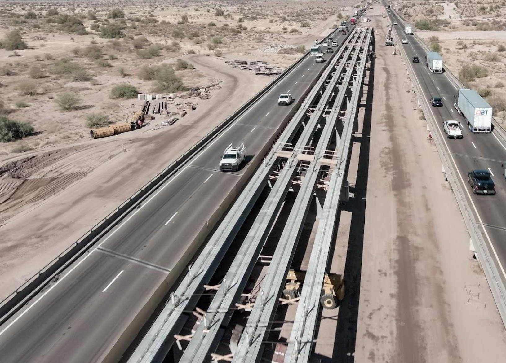
Construction of bridge girders for the Gila River on I-10 in Pinal County
