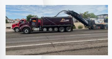
the concrete pavement and repair areas that are cracking or beginning to break before final roadsurface treatments are applied.
