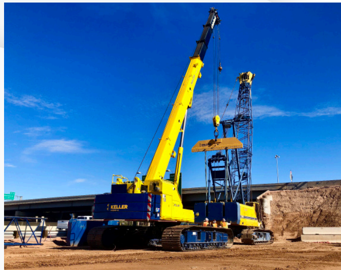
Crews assembled cranes in preparation for the drilled-shaft foundation installation at the 48th Street bridges over I-10.
