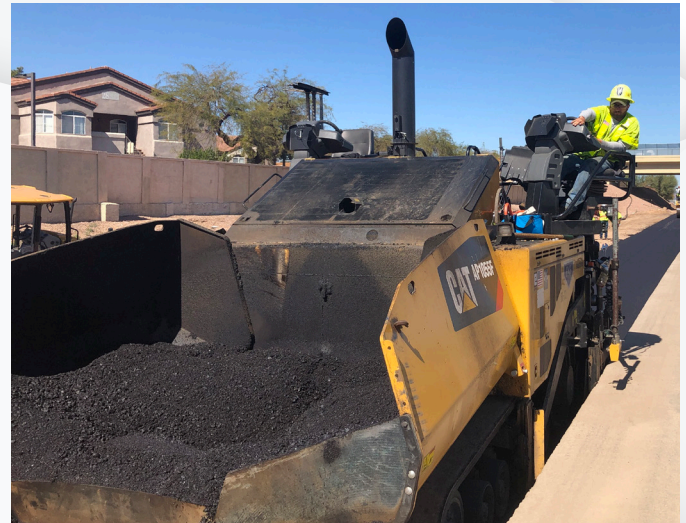
Crews place asphalt pavement as the base layer of I-10 south of Guadalupe Road. Next, workers will place concrete pavement on the asphalt. Rubberized asphalt will be the top layer in the East Segment of the project.
