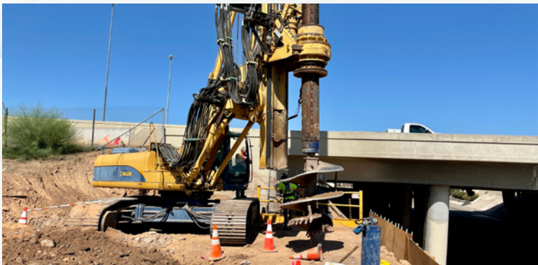
Workers drill shafts for the foundation of the new Collector-Distributor road bridge over Southern Avenue.
