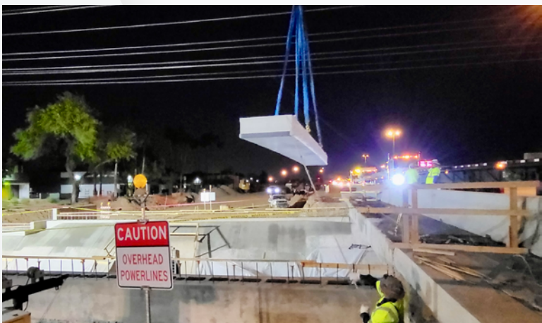
Workers place the 48th Street bridge beam near Medtronic Way. The beam weighs approximately 40,000 pounds.
