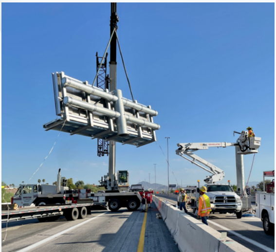
Workers place a DMS for eastbound traffic on I-10 between Baseline and Guadalupe roads.
