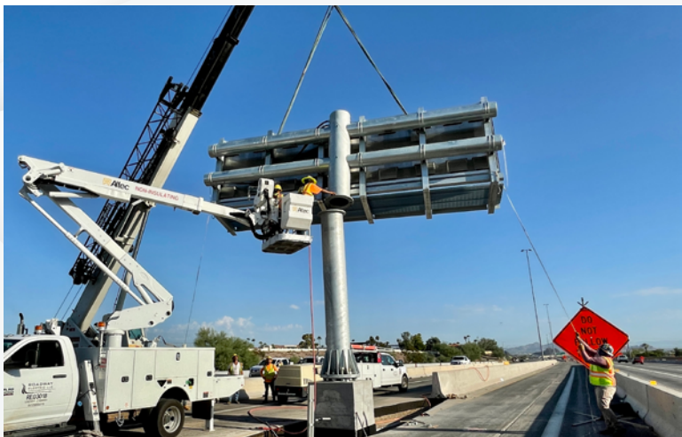
Workers place a DMS for eastbound traffic on I-10 between Baseline and Guadalupe roads.
