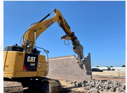
A crew removes a wall to make room for construction of the new westbound CD road.
