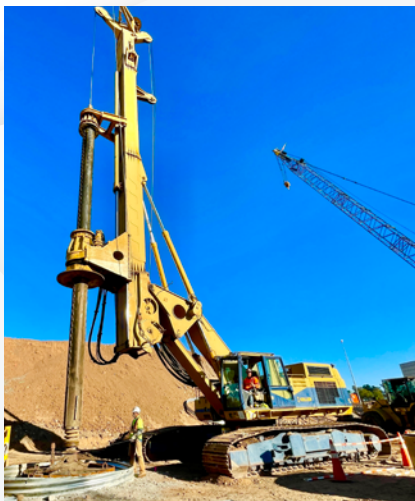
These drilled shafts are 10 feet wide and approximately 70 feet deep.
