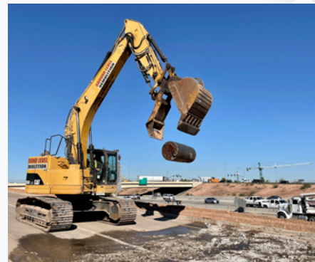
As part of the ramp reconfiguration, crews break up the pavement of the eastbound I-10 on-ramp at northbound 40th Street.
