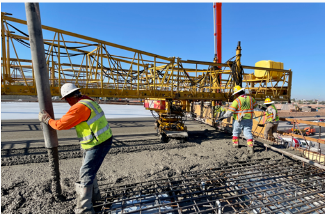
Crews place the deck for the new Broadway Road bridge over I-10 using a bridge paving machine called a Bid-Well.
