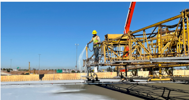
Workers spray curing compound on the finished concrete to lock in moisture as the concrete hardens and gains strength.
