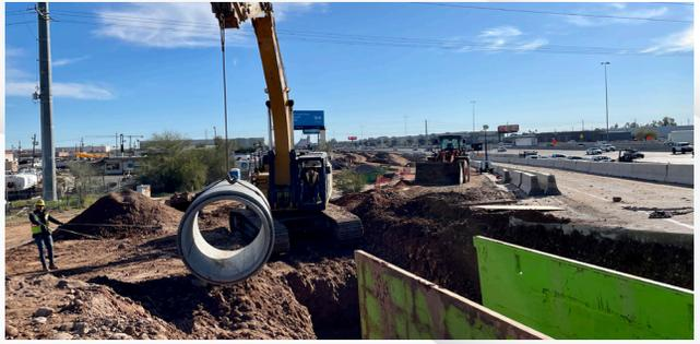
As part of the ramp reconfiguration, crews relocate storm drain pipe under the westbound I-10 off-ramp at 32nd Street.
