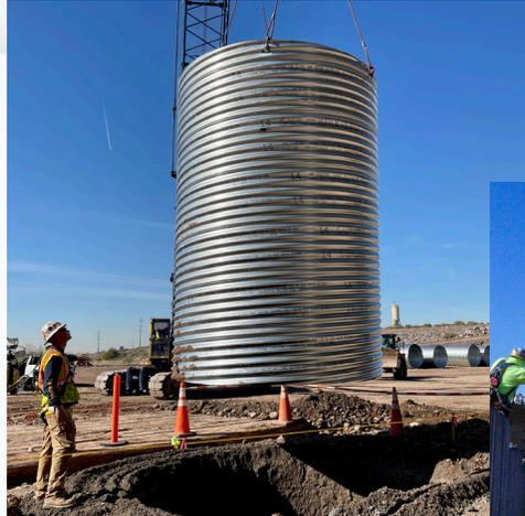
*A crew uses a crane to install a drilled-shaft foundation liner for the bridge that will widen eastbound I-10 over the Salt River.*
