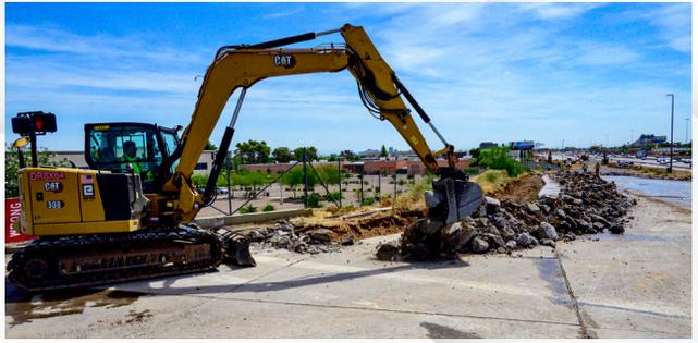
Workers remove the westbound I-10 off-ramp at 40th Street pavement to reconfigure the ramp and make room to widen I-10.
