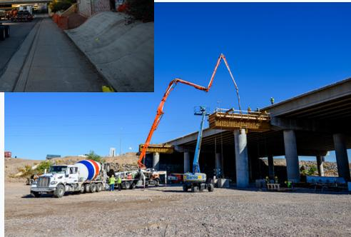
A concrete pump fills a pier cap form to widen the eastbound I-10 bridge over the Salt River.
