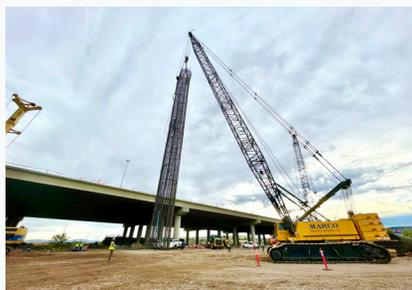
*A crew uses a crane to install a drilled-shaft foundation rebar cage for the bridge that will widen eastbound I-10 over the Salt River.*
