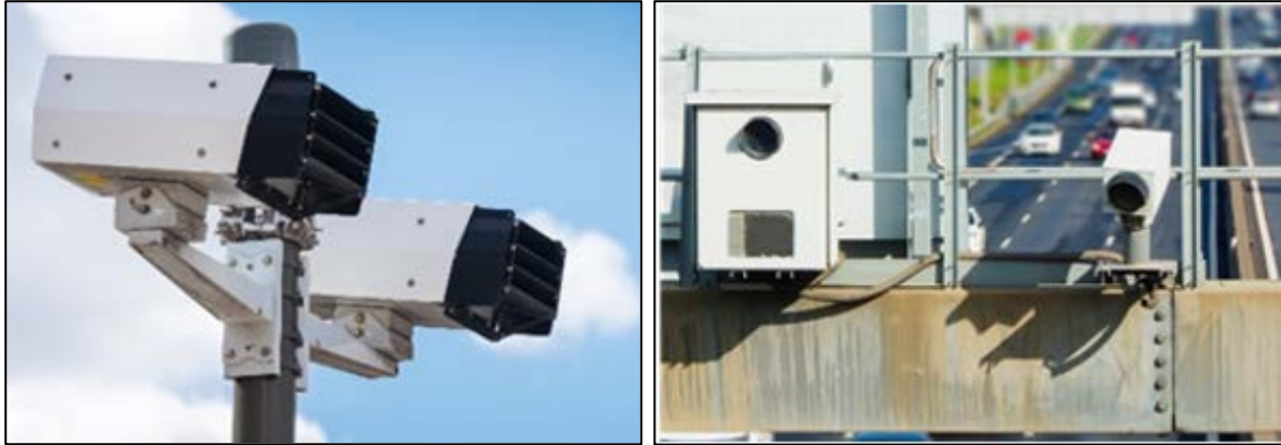
Figure 5-12. CCTV Camera and Radar Detection for TPAS
