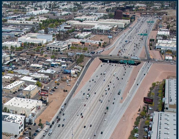
*Crews reconfigured the I-10 interchanges at 32nd and 40th streets, which included removing the loop ramp that connected southbound 40th Street to eastbound I-10.*
