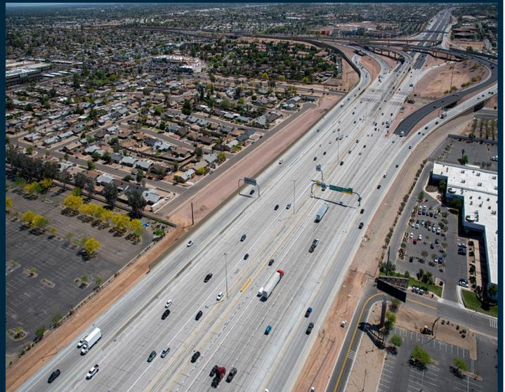
*Crews constructed the westbound CD road between Baseline Road and 40th Street to separate through-traffic on I-10 from local traffic entering or exiting the highway.*
