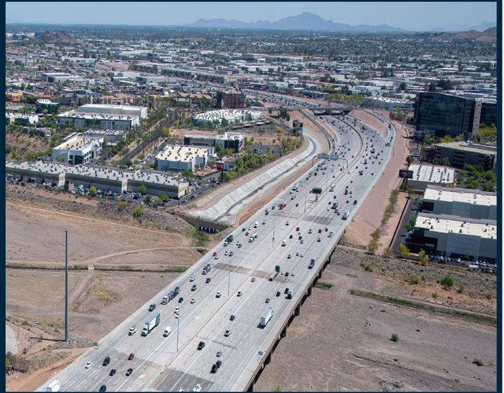
*Crews widened the I-10 bridges over the Salt River to make room for six general purpose lanes and two HOV lanes in both directions.*
