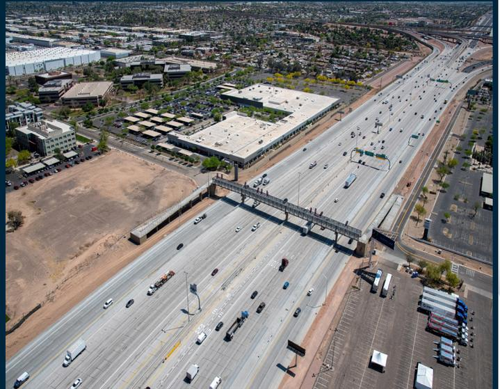
*Crews constructed two new multiuse bridges, one at Alameda Drive and one at the Western Canal, to provide safe new crossings for pedestrians and cyclists over the freeway.*
