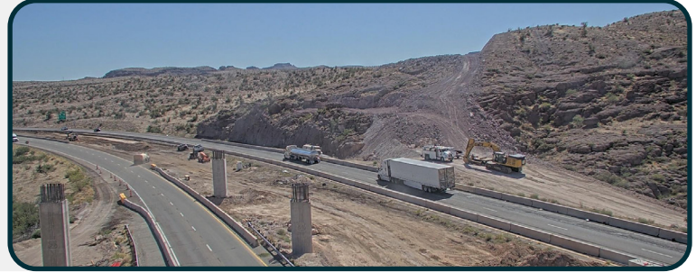
Bridge shafts are being drilled and bridge columns and pier caps are being installed along I-40.
