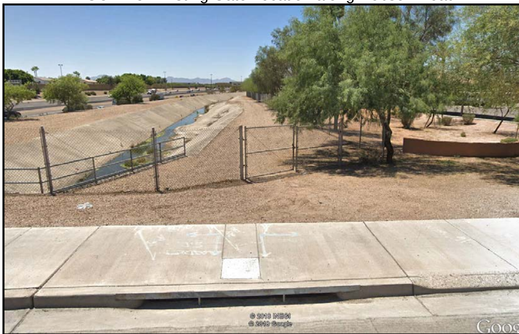
FIGURE 5. Existing Gate Location along Dobson Road
