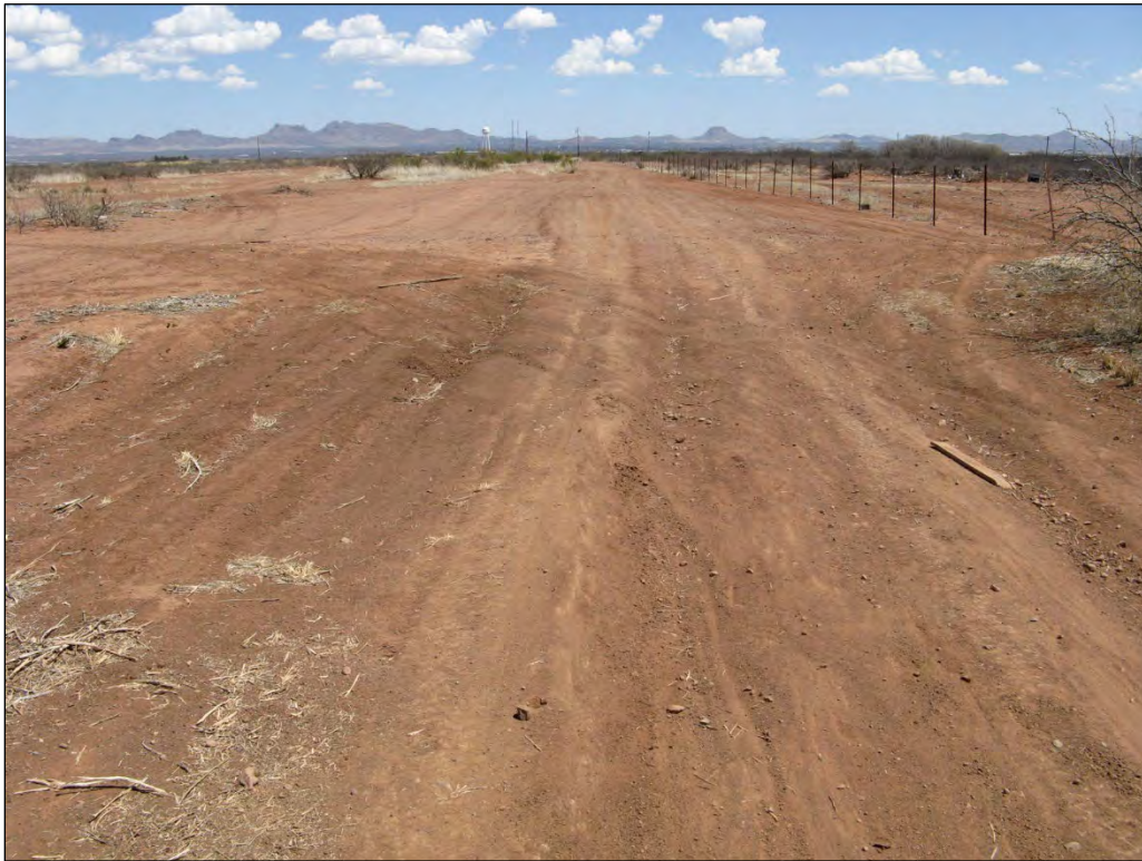
Photo A-5. East view of gas line from the northwest corner of Alternative 2.
