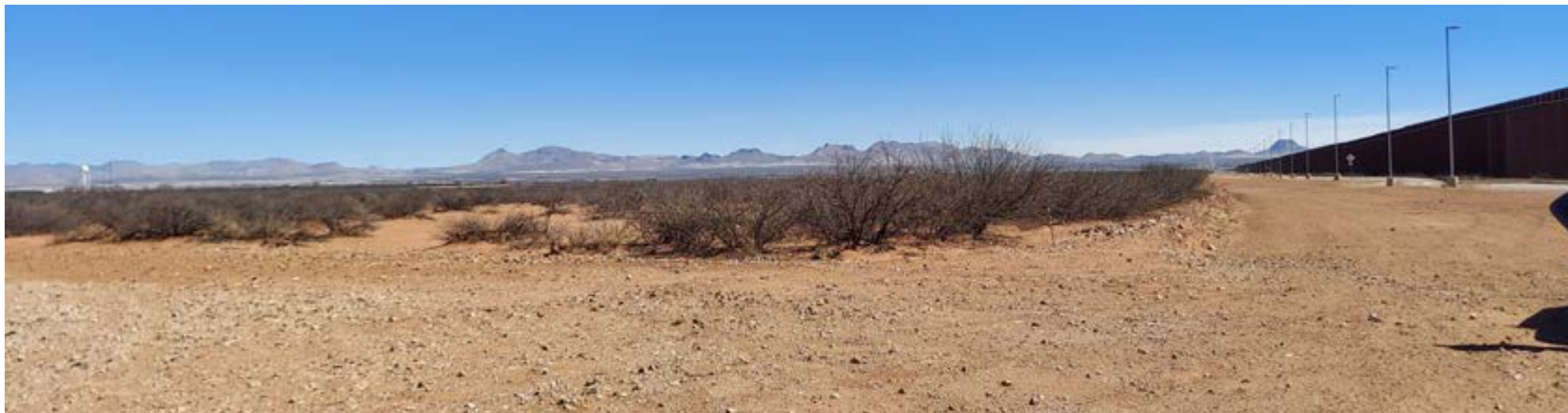
Figure 23. WB view along International Avenue showing wide, flat landscape with border wall in the middle ground and mountains in the background.
