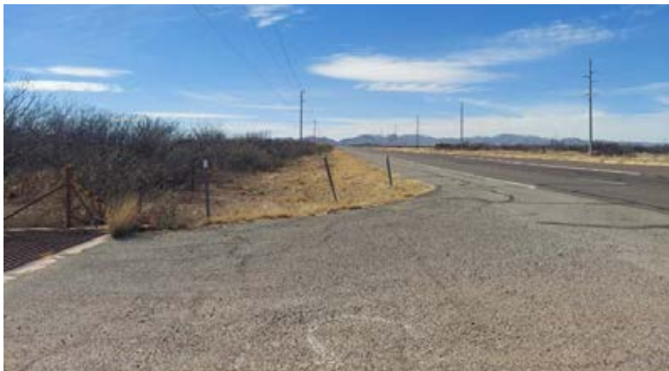
Figure 11. WB view showing flat FG along Hwy 80 and JRR intersection.
