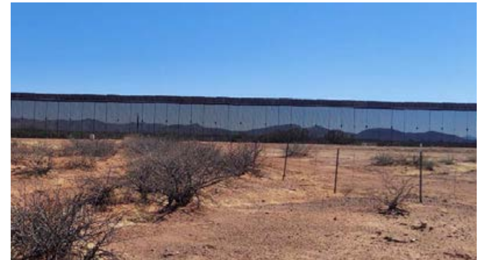
Figure 44. SB view showing a barbed wire fence adjacent to unpaved roadway.
