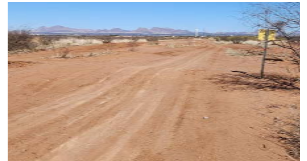
Figure 28. EB view on Puzzi Ranch Rd, the City of Douglas is visible in the BG.
