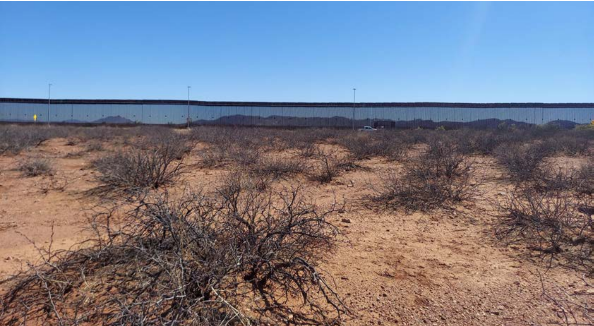
Figure 34. SB view showing the flat foreground with the prominent border wall.
