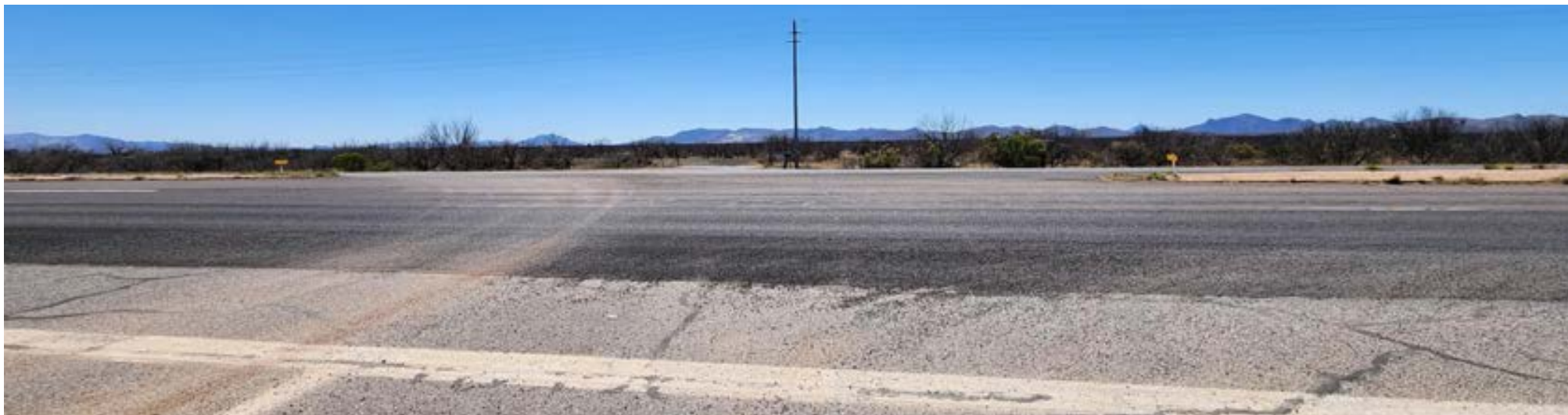
Figure 40. SB view showing the Highway 80 structures in the foreground.
