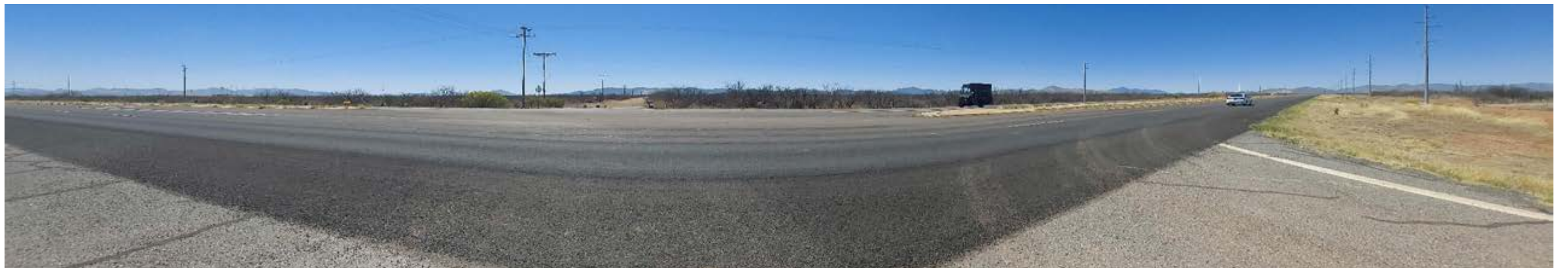
Figure 9. Panoramic view showing east, south, and west views along the JRR alignment, south of Hwy 80.
