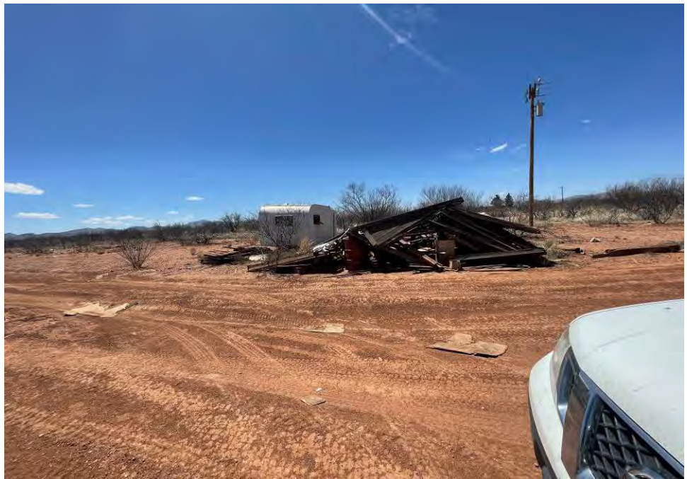
Photograph 17: View of construction debris near James Ranch Road on the eastern portion of the Project Area
