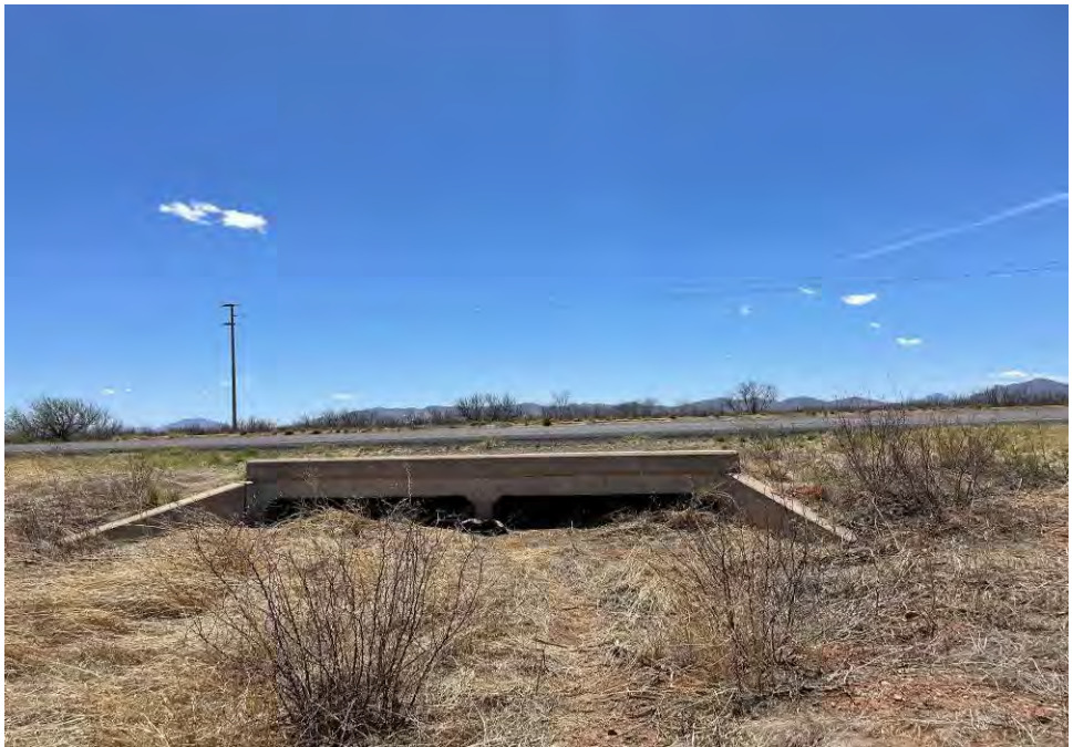
Photograph 10: View looking south at a stormwater culvert along State Route 80.
