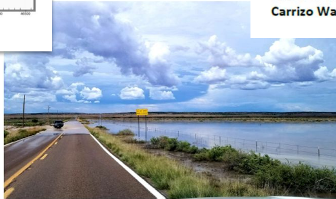
Roadway overtopping at around Sta. 432+00 South of Existing Box Culvert.
