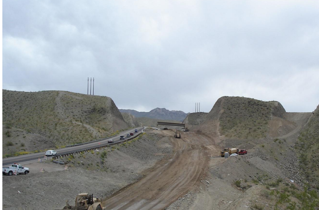
US 93 Two Lanes to Four Lanes
