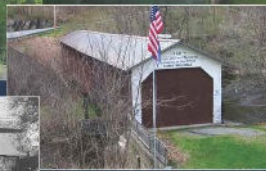
▲ The Redleigh Covered Bridge is the last remaining American wooden bridge that has cast iron "shoes" incorporated into its design. This feature was patented by K. Corning of Troy, New York. Photo courtesy of Town of Salem Historian.
