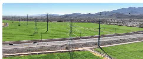
SRP-T, APS, and WAPA Overhead Power Lines
