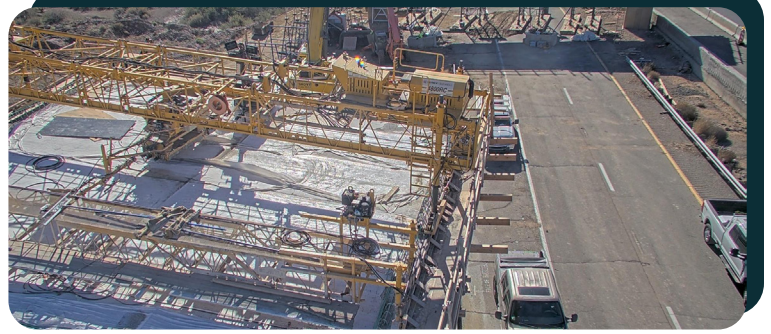
Work on the south-to-east flyover bridge deck along I-40 continues.
