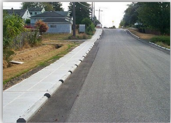
Figure 8 | Curbing with drainage cuts. Example of curbing with breaks to allow drainage while providing separation from roadway.
