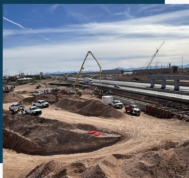
Kino Parkway Abutment Wing Wall - Crews are pouring concrete for the north wing walls of the new Kino Parkway bridge over I-10. Wing walls help hold back soil and support the roadway as it approaches the bridge.
