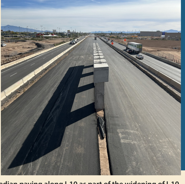
Median paving along I-10 as part of the widening of I-10.
