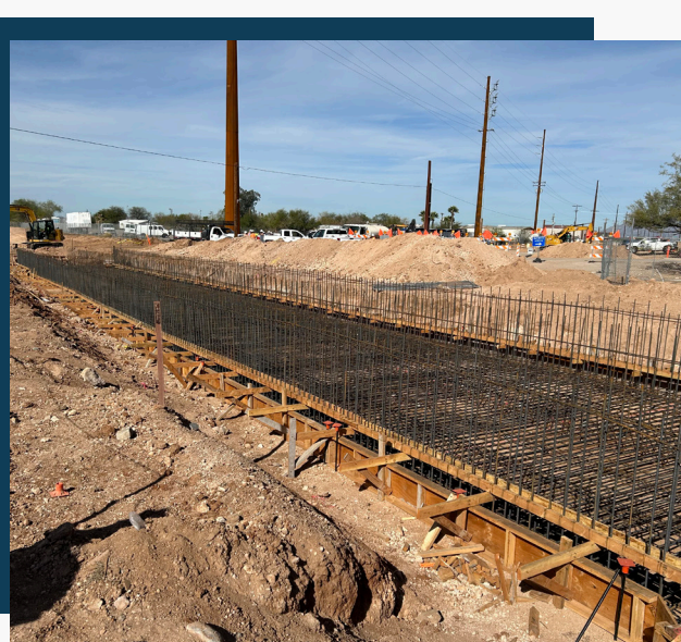
Country Club Road Box Culvert - Crews are building the floor of a concrete drainage structure. Wooden forms and steel reinforcement are in place to shape and strengthen the concrete. The next step is to pour the concrete. Once the concrete hardens, the forms will be removed and construction on the side walls will begin.
