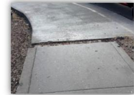
Figure 1 | Bullion Plaza Cultural Center and Museum. A segment of sidewalk a joint gap and uneven widths.
