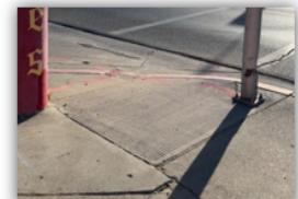
Figure 2 | Miami Ave/US 60 Intersection. A curb ramp with limited ramp width and no ADA-compliant detectable warning surface.
