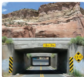
The area's intact sandstone and siltstone will likely provide excellent support for bridge foundations.
