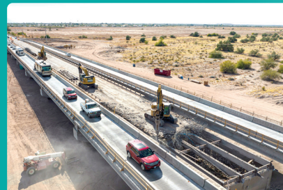
SR 79 GILA RIVER BRIDGE CMAR
