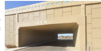
Exhibit 8: Davis Avenue Closed Concrete Frame Structure
