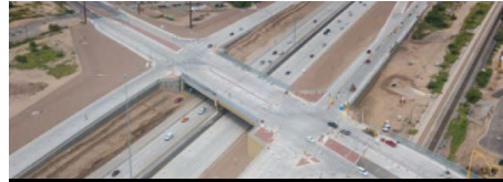
I-10 Ruthrauff Road Traffic Interchange
