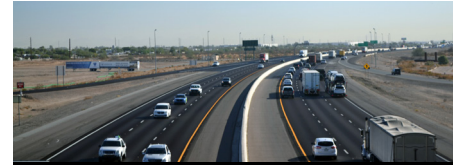
I-10, SR 85 to Citrus Road HOV/GPL Widening
