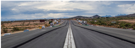
I-10, Earley to I-8 GPL Widening
