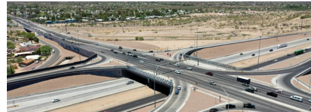
I-19 Ajo Way Traffic Interchange
