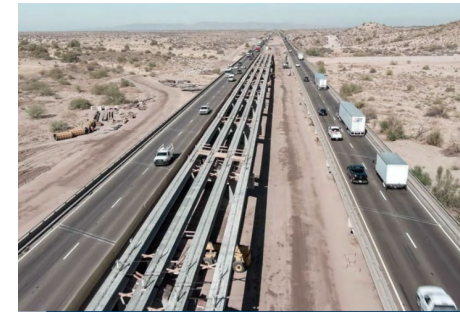
Construction of bridge girders for the Gila River on I-10 in Pinal County
