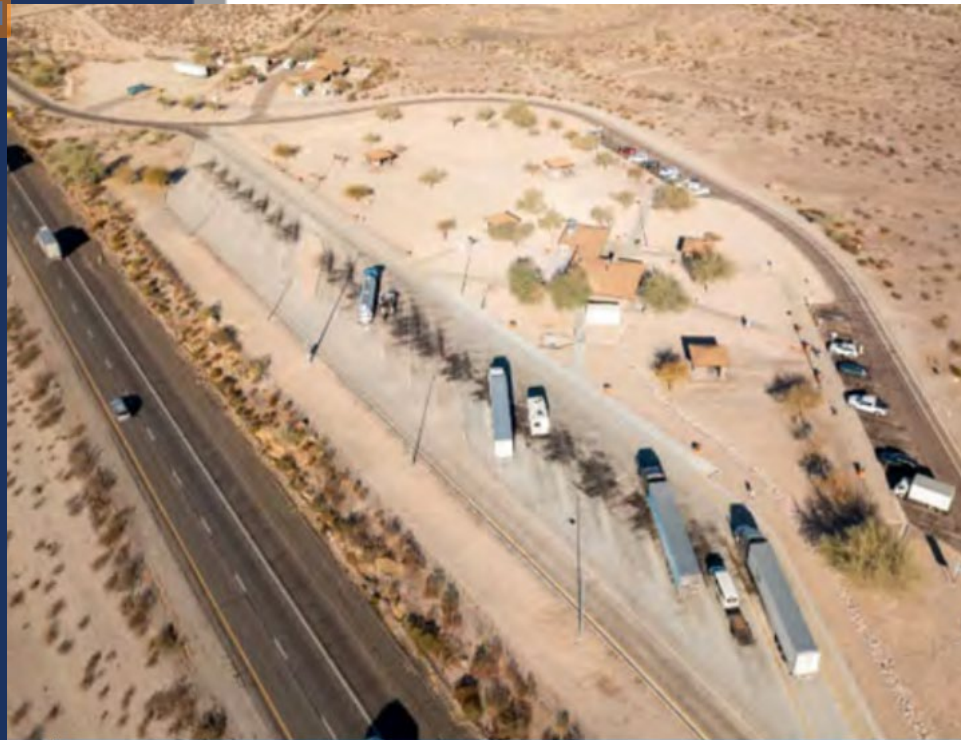
Bouse Wash Rest Area on I-10 in LaPaz County
