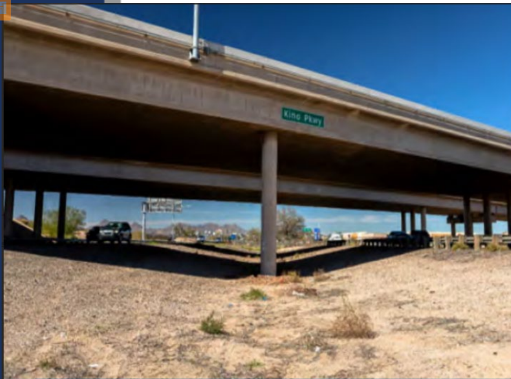
Kino Parkway overpass on I-10 in Tucson
