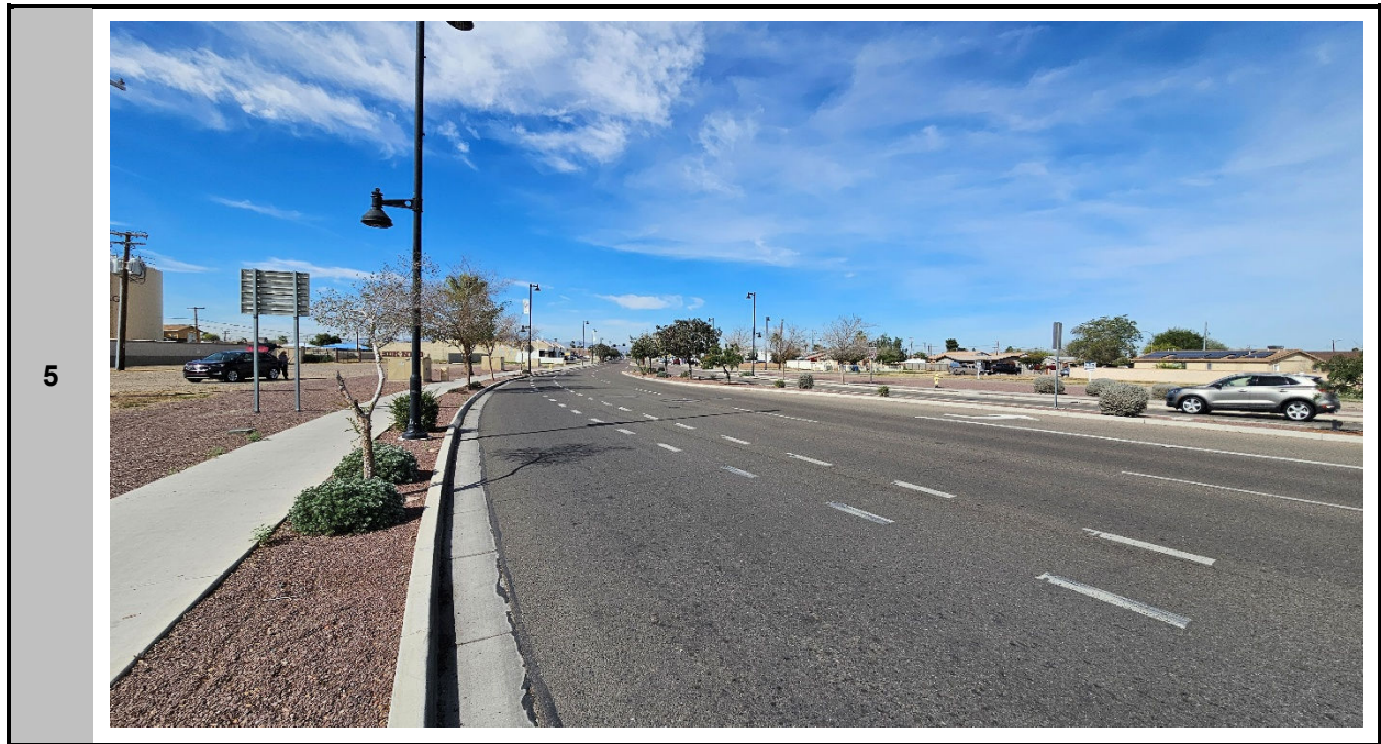
View west along Thunderbird Road (subject property on left)
