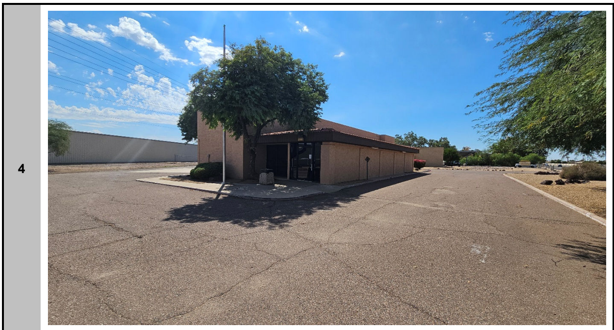
View southeast toward the subject building
