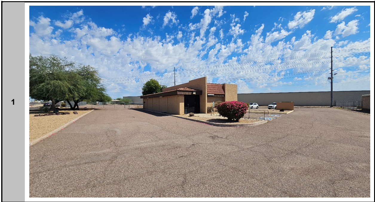
View northeast toward the subject building
