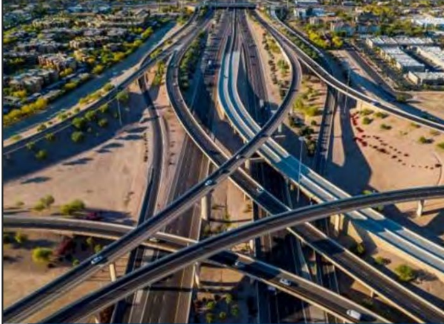
The Broadway Curve on I-10 in Maricopa County
