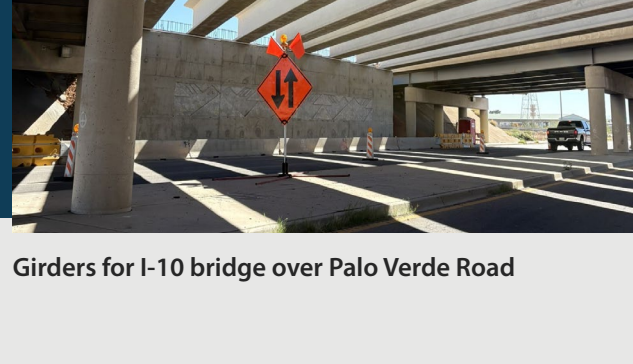
Girders for I-10 bridge over Palo Verde Road
