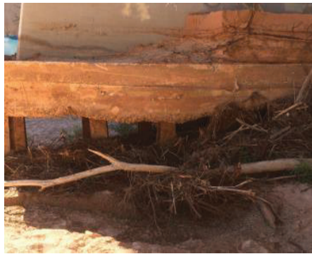
Figure 3-6 | Scour at a Bridge Pier
