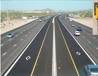
Arterial Street Widening
