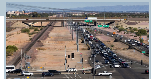
US 60 (looking east): NB SR 303L to WB US 60 to NB 163rd Avenue (PM) is one of the two heaviest movements through the TI. The inverse the other heaviest movement.
